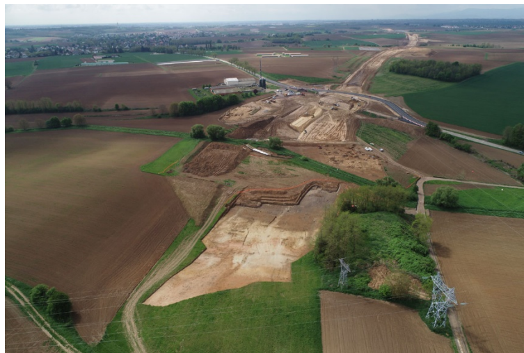
Aerial view of site 5-8, Excavation 5-8 of the Western Strasbourg Bypass, Kolbsenbach Valley, Truchtersheim. Shot: Drone Alsace, 2019
